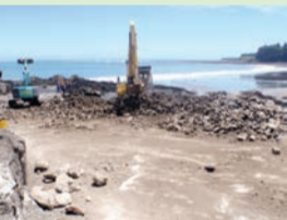
At Middleton's Bay Ramp upgrade. Another example of Coastal 'can do'. See page 18.
